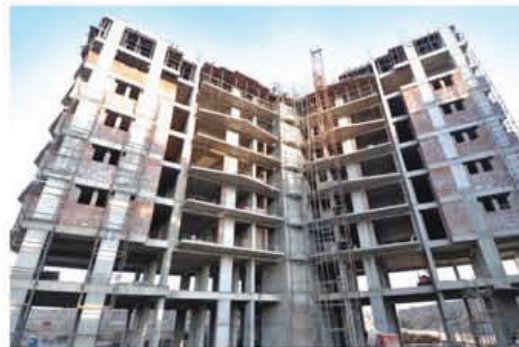
MACEO, SECTOR-91, GURGAON
