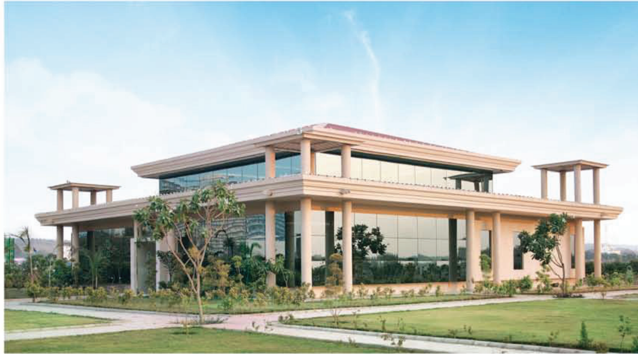
ACTUAL PICTURE OF THE ESTATE PREVU, MARKETING OFFICE AT THE ANANT RAJ ESTATE SITE
