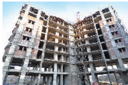
MACEO, SECTOR-91, GURGAON
