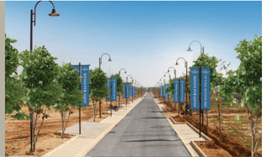
road infrastructure in progress >
