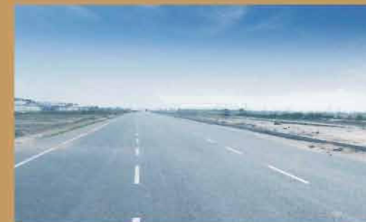
AN ACTUAL PHOTOGRAPH OF DWARKA EXPRESSWAY
