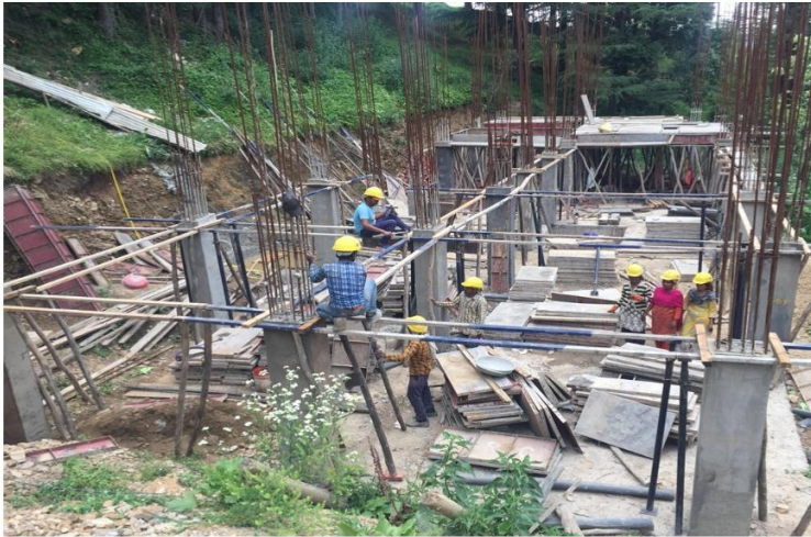
Formwork of Block B ground floor is in progress
