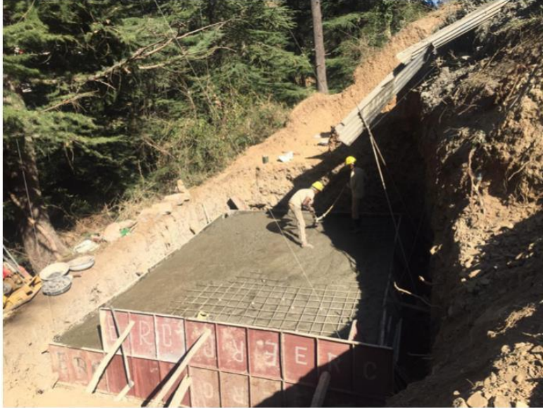
RCC band casting of retaining wall
