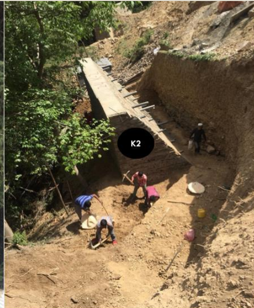
Manual excavation for Retaining wall in front of Block J-K
