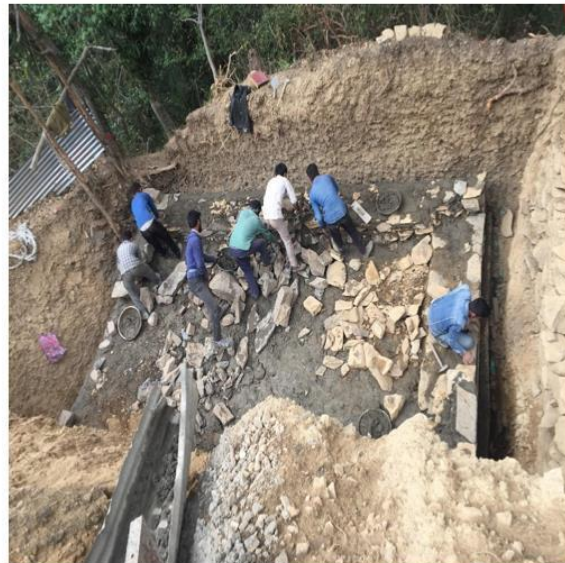
Stone work & rcc band of retaining wall in front of block C
