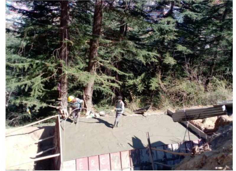
1:3:6 concrete filling in voids
