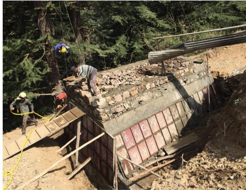
Stone work of retaining wall
