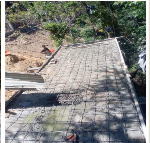
Reinforcement binding work for RCC Band of Retaining Wall
