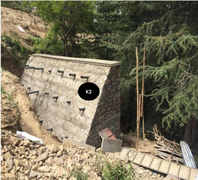
Retaining wall K2 in front of Block J-K
