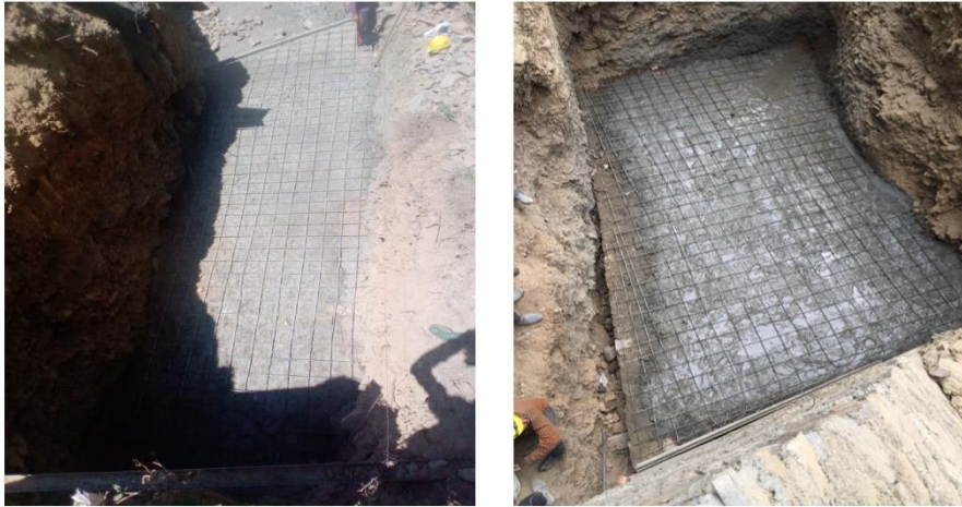
Binding of reinforcement of RCC Band
