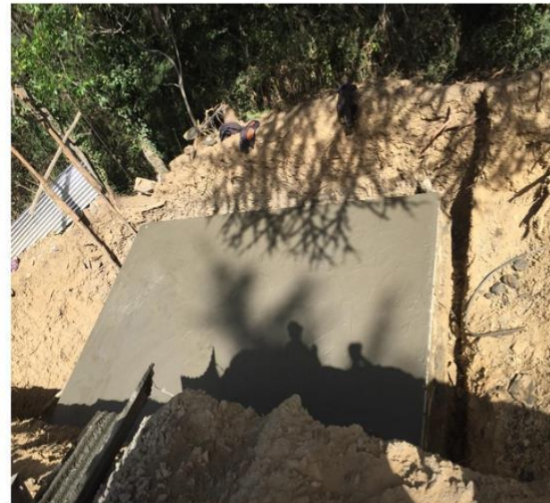
Stone work & rcc band of retaining wall in front of block C
