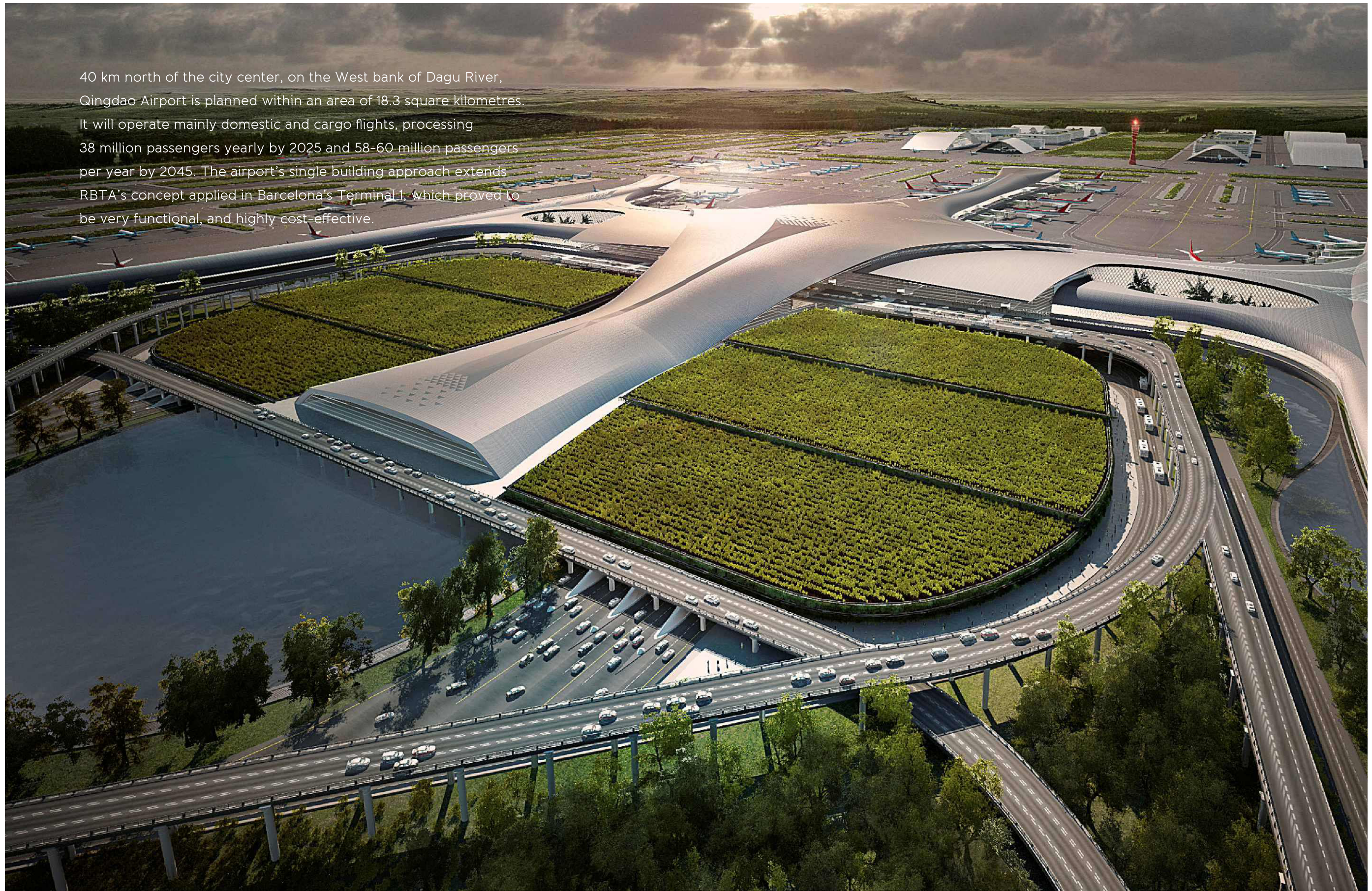
Qingdao New Airport, China
