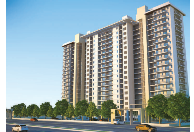
UNDER CONSTRUCTION GRAND CENTRA Sector 37 C, Gurgaon
