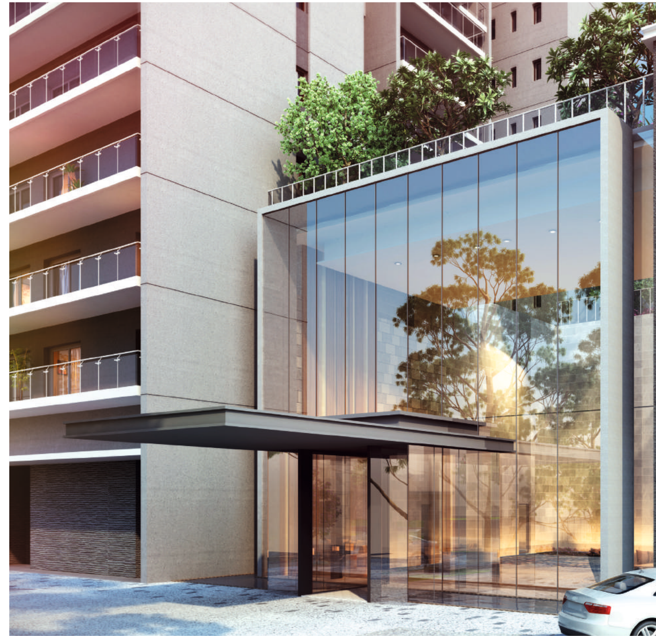
Tower C Drop-Off •
