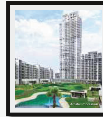
M3M golfestate Fairway WEST GOLF COURSE ROAD EXTENSION SECTOR-65, GURUGRAM
