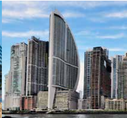
Trump International Hotel & Tower Panama City, Panama
