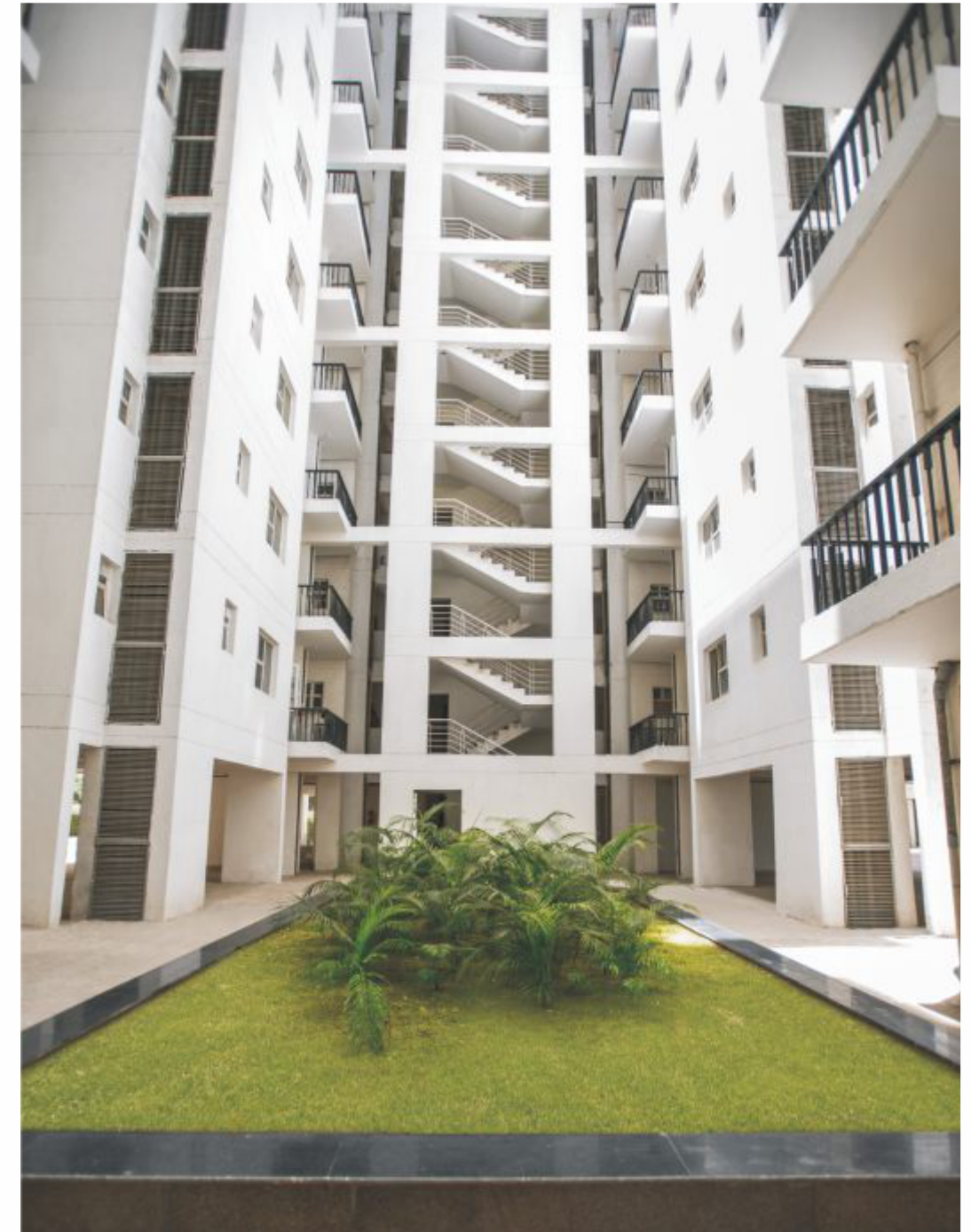
INTERIOR LANDSCAPED COURT OF ASTER COURT
