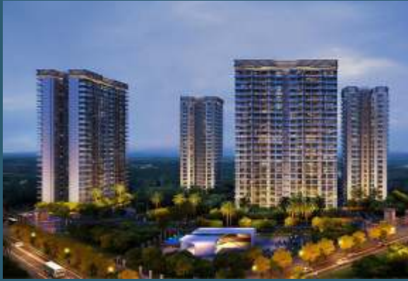
PARAS DEWS, DWARKA EXPRESSWAY
