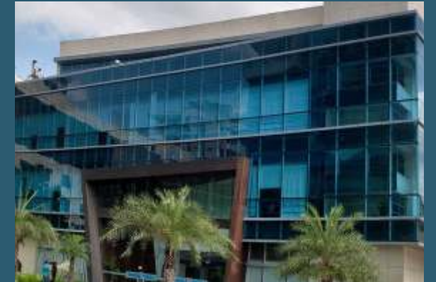
PARAS TWIN TOWERS, GURUGRAM
