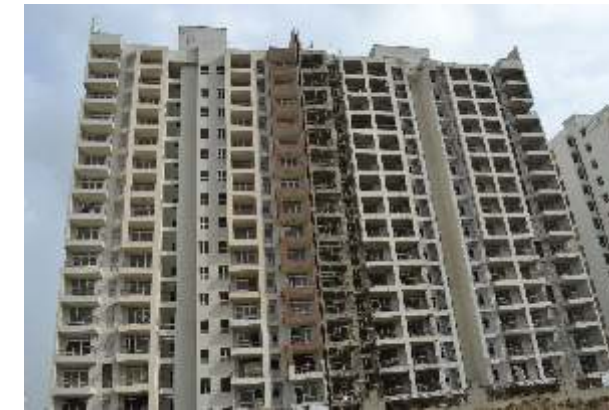
Navodaya - construction photograph
