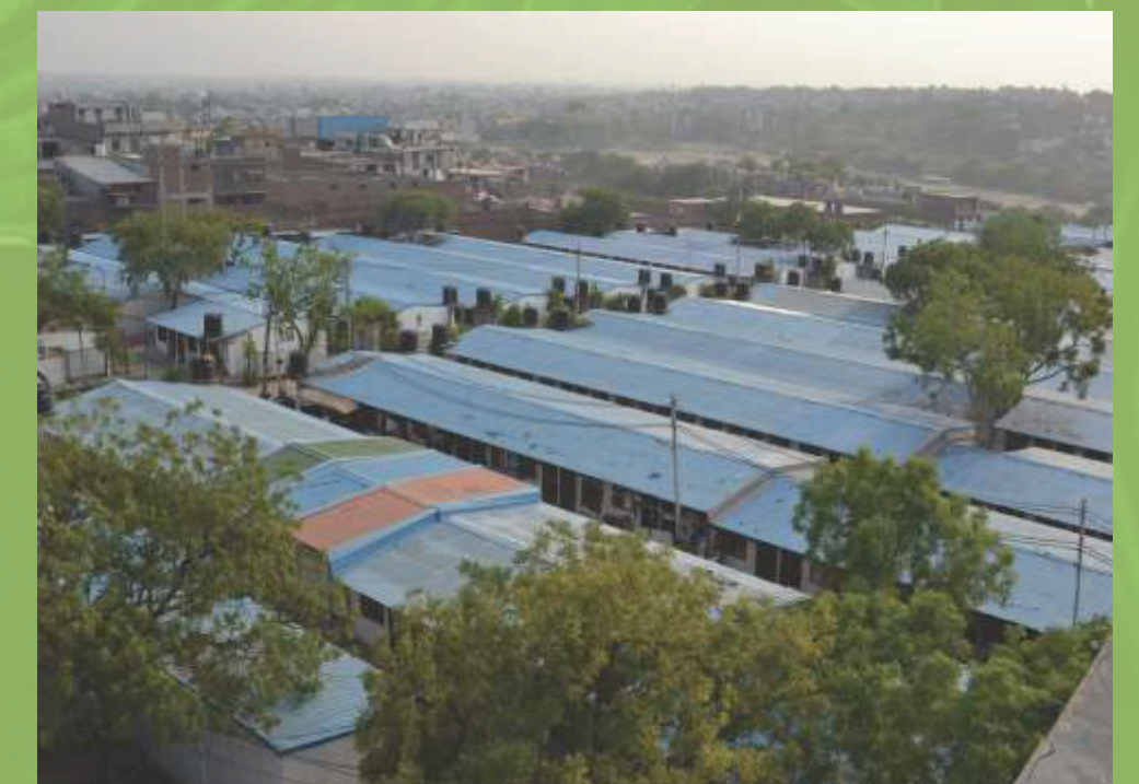
First of it's Kind In-Situ Slum Rehabilitation Scheme at Kathputli Colony
