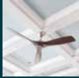
CEILING ACRYLIC EMULSION PAINT/ OIL BOUND DISTEMPER
