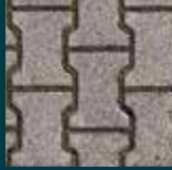
INTERNAL ROADS INTERLOCKING BLOCKS/ TREMIX CONCRETE ROAD
