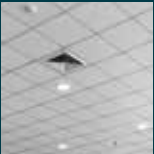
CEILING GRID FALSE CEILING
